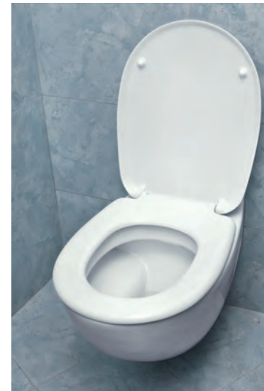
Marked surfaces prior to cleaning
